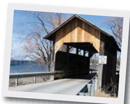
39 ft (approx 12 m) Lakeshore Bridge spanning Holmes Creek.
